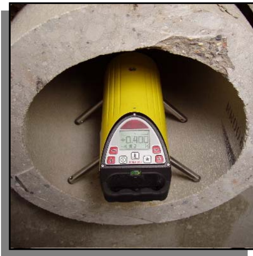
Inside the Pipe
